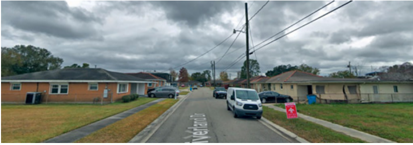
Figure 12 Typical Chalmette street.
