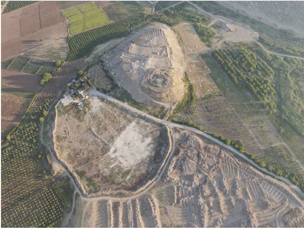
Figure 7. Aerial photograph showing the bulldozing work at the Ain Dara site (Ammar Kannawi/SIMAT 2021).
