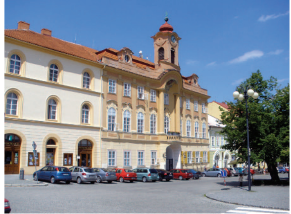
Figure 7. Town Hall in Čáslav: Jan Josef Wirch led the Baroque reconstruction of the original Gothic Town Hall, 1765–1769. Its Memorial Hall contains Žižka's remains.
