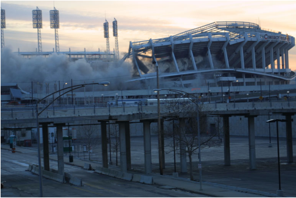
Figure 1. Cinergy Field (formerly Riverfront Stadium) imploding, December 30, 2002, photograph by Shelby Bell.
