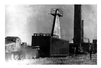
**Fig. 9.** The mobile drilling shelter PBU-3 installed above the mouth of hole No. 3G (summer season of 29th SAE, 1984).
