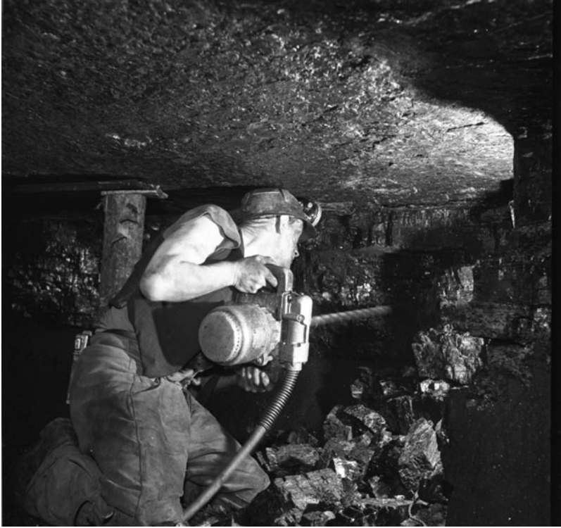
Figure 1. Miner drilling the coalface. (Photograph courtesy of the National Coal Mining Museum for England).
