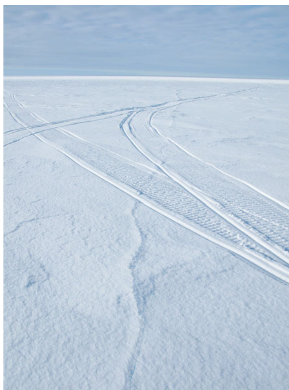
Fig. 2. Surface expression of a strand crack in the strain grid, near e2 as shown in Figure 3. Snowmobile tracks crossing the fracture are ~0.38 m wide.
