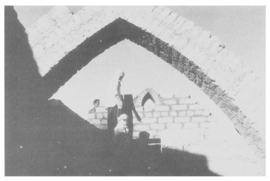
Newly introduced adobe construction techniques are solving housing problems without increased destruction of trees and thatch for roofing materials ( $John\ Newby/WWF$ ).
