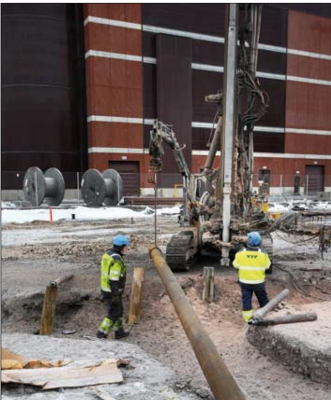
*The pile casing, a drilling pipe during installation, and part of the load-bearing pile structure.*
