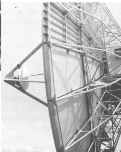
Backstructure of 20 m radiotelescope
