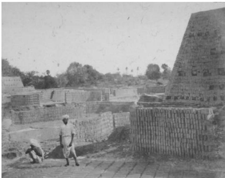
Figure 2. Clamps along the Hooghly river, near Calcutta, ready to be dismantled (right and left), with, in the foreground, stacks of green bricks drying, on which two workers are standing. Hand-coloured photographic print by Frederick Fiebig (c.1851–1852).
