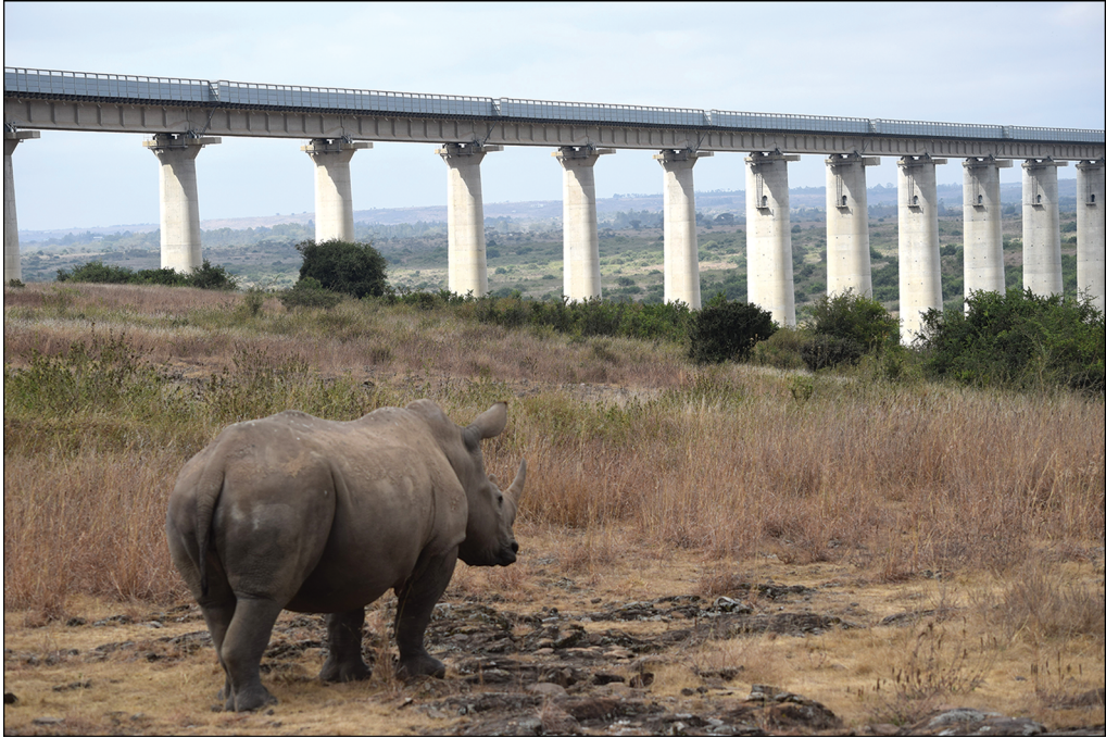
Figure 4. A viaduct passing through the Nairobi National Park, part of the 600km-long railway built with Chinese finance and completed in 2017 to connect Mombasa with Nairobi and Suswa, Kenya. Photograph by R. Witcher.
