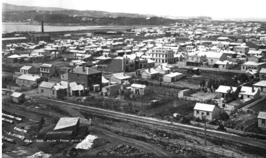
Figure 2. The Flat from the Hillside. This photograph was taken of the most densely populated part of Caversham Borough just before the beginning of the period studied. As can be seen, the area was dominated by a small number of two-storied buildings, usually shops or workshops, and a lot of small cottages situated on their own plots of land. The gasworks, the railway workshops, a substantial brick works and a flourmill dominated this part of the Borough and manual workers inhabited the cottages.
