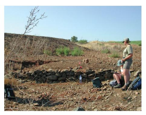
**Figure 7.** Check dam at Potami Strata Oritissas, trapping cobbly sediment in a shallow gully incised through Pleistocene pediment, July 2003. Soil colour 5YR 3/4. (Photograph: Jackaline Robertson.)
