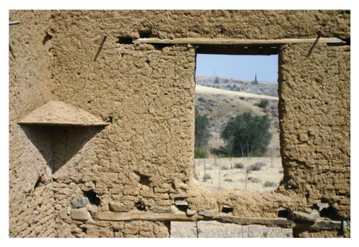
**Figure 8.** *Mandres: interior of house looking northwest, with shelf made of threshing sledge plank (left), upper floor doorway, sockets for beams, mud bricks (below) and mud plaster (above), June 2016. (Photograph: Michael Given.)*
