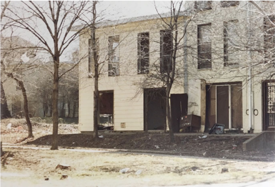
Figure 6. Abandoned buildings at LaCledde Town, c. early 1990s. SHSM/John C. Danforth papers (unprocessed), box 197.
