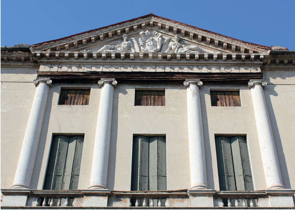
9. Villa Pisani, south facade, detail of Ionic order and pediment. Photo: author
